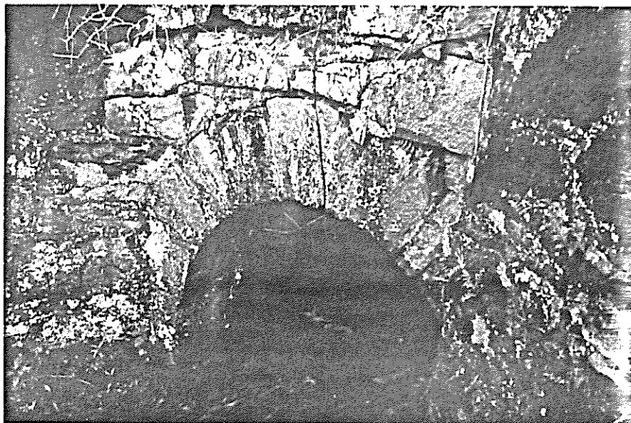
Key Stone Arch in a Culvert
