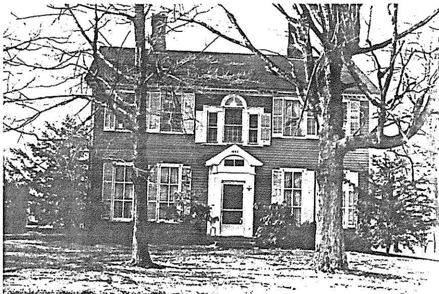
Georgian farmhouse, ca. 1803.
