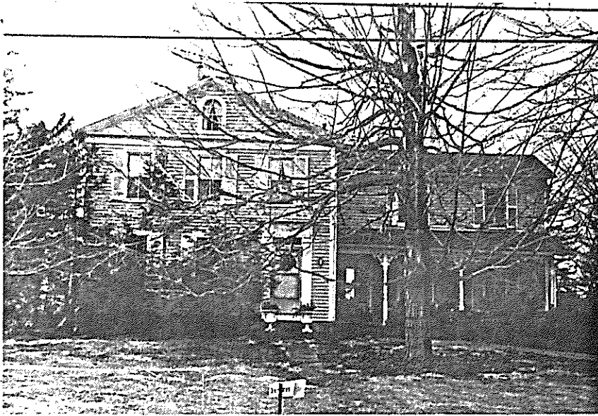
33A. Federal farmhouse (1820's) added onto earlier Georgian structure. House site of Stephen Heaton, ca. 1745.
