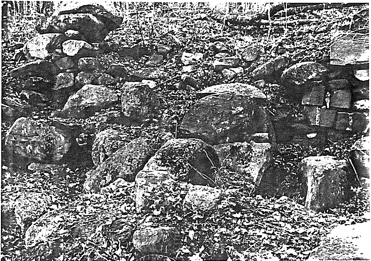
Foundation of Grist Mill
